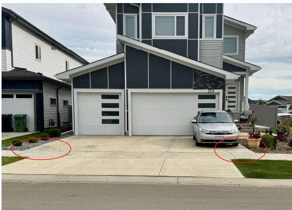
Homeowner filled in driveway curve with concrete
